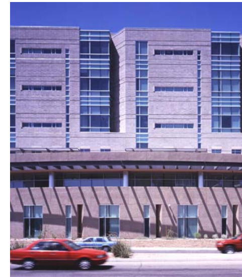
Minimize solar gain with dominant ratio of solids to void in building mass
